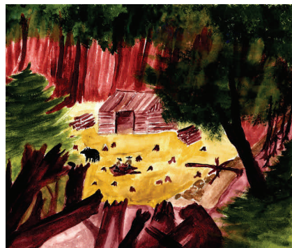
Eight men and a team of oxen could put up a cabin in a day—up to the roof.
